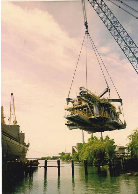
Abb. 5: Entladung am Pier in Detroit
