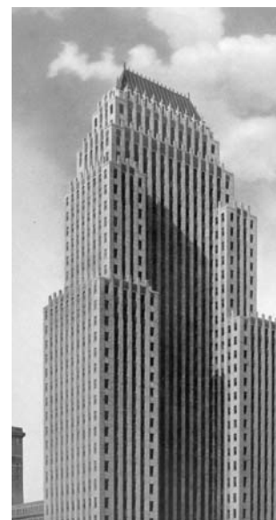
Koppers Building in den USA
