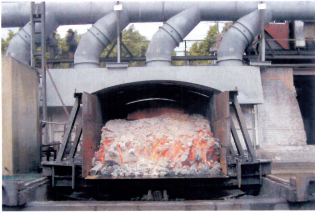
Hot coke being pushed into the hot car to take it to the quench tower
